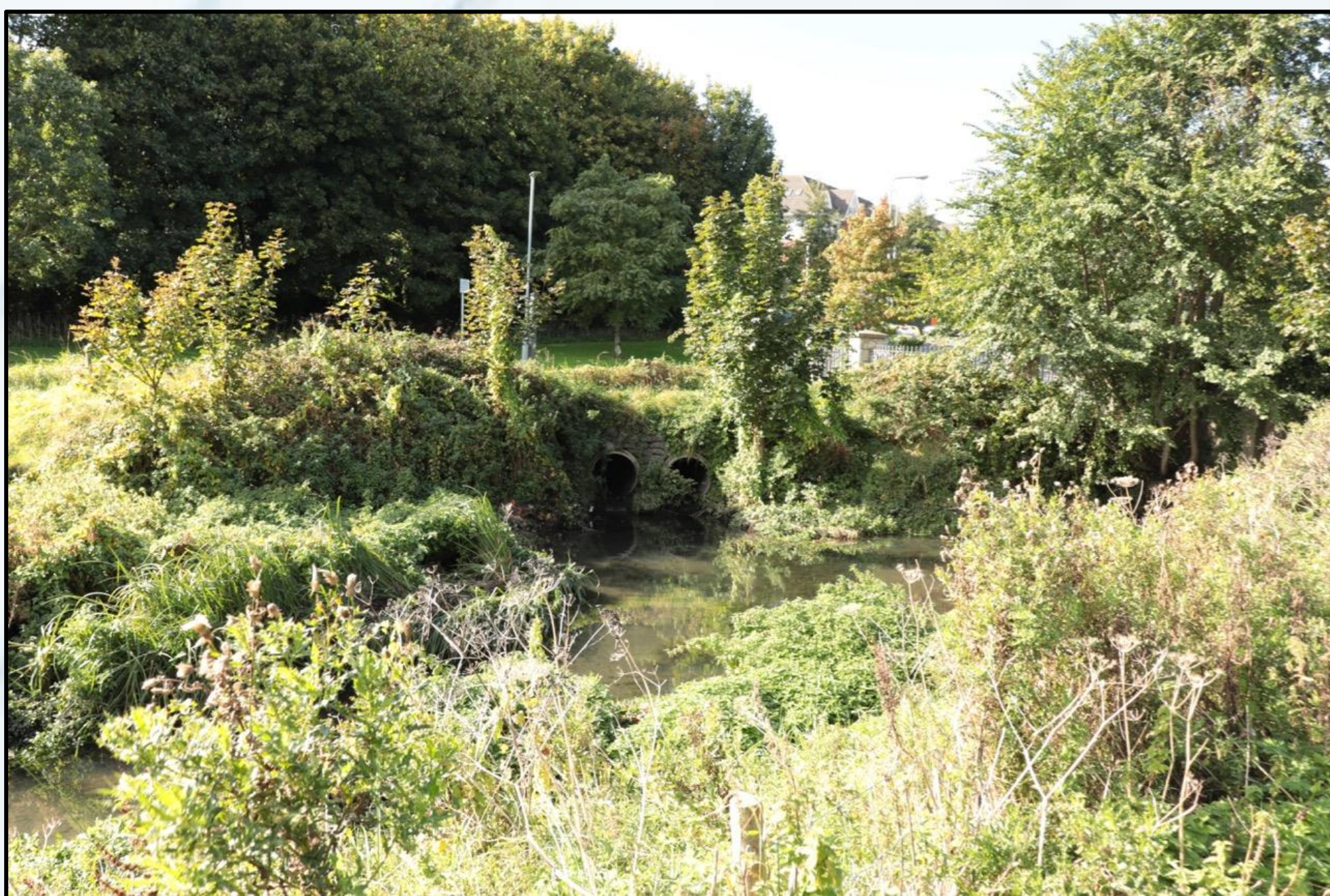
Existing 1050mm dia. Pipes
